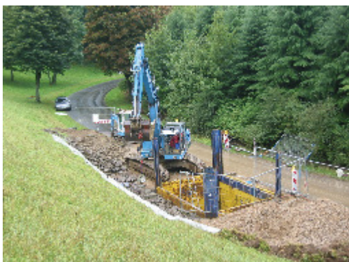
Fig. 5: Test pit on the downstream toe
