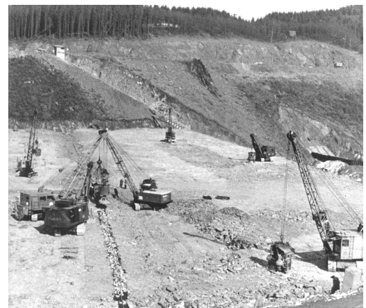
Fig. 4: Compaction with a crane vibration unit
